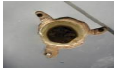
Cut around drain
