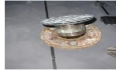
Seal and install drain
